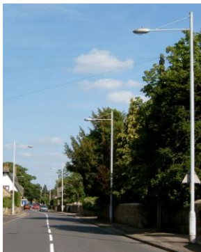
Trunk road style highway lights
